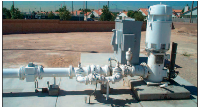
Las Vegas Valley Water District, Nevada, operates the largest ASR wellfield with 42 ASR wells. Total recovery capacity is 157 mgd.
